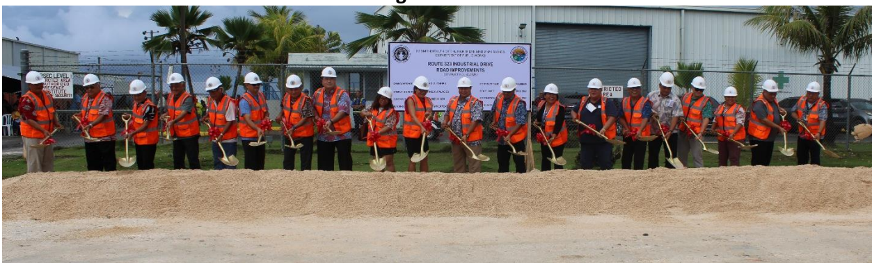
Pictures above, Route 323 Industrial Drive road improvement (Seaport area) project Contract amount ($1,305,988.00) funded by FHWA.
