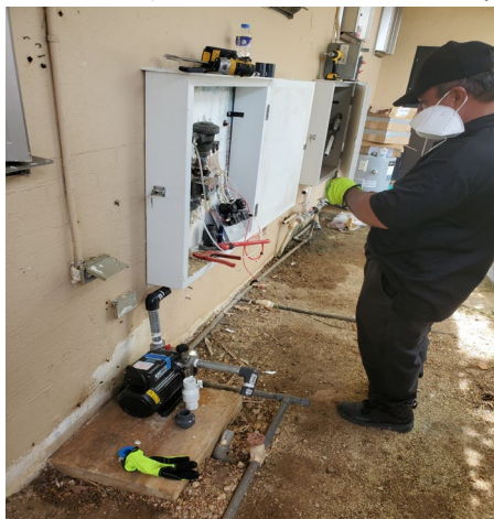
Electrical Repair of Tinian Detention Facility
