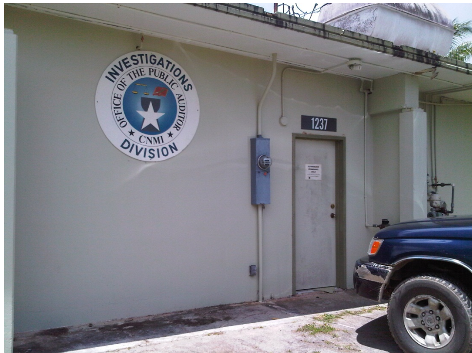
Investigation Unit office building
