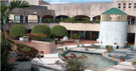
Relocated CUC Offices at former La Fiesta Mall
