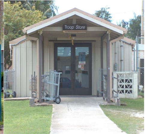
AAFES Troop Store located at the Army Reserve Facility
